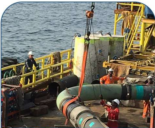
Offshore Pipe Laying Operations
