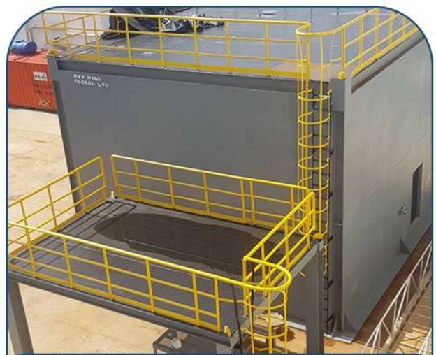
Fabrication and Installation of Workshop on Milaha barge at Onne
