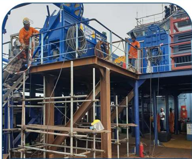
Kalaface Deck Extension Project at ONNE FOT
